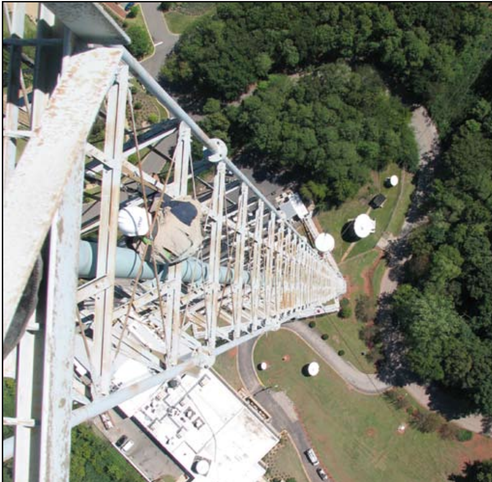
Inspection of a 1000 foot Guyed Tower
