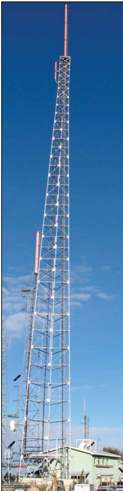
Self-Supporting Towers at Mt. Wilson, CA
