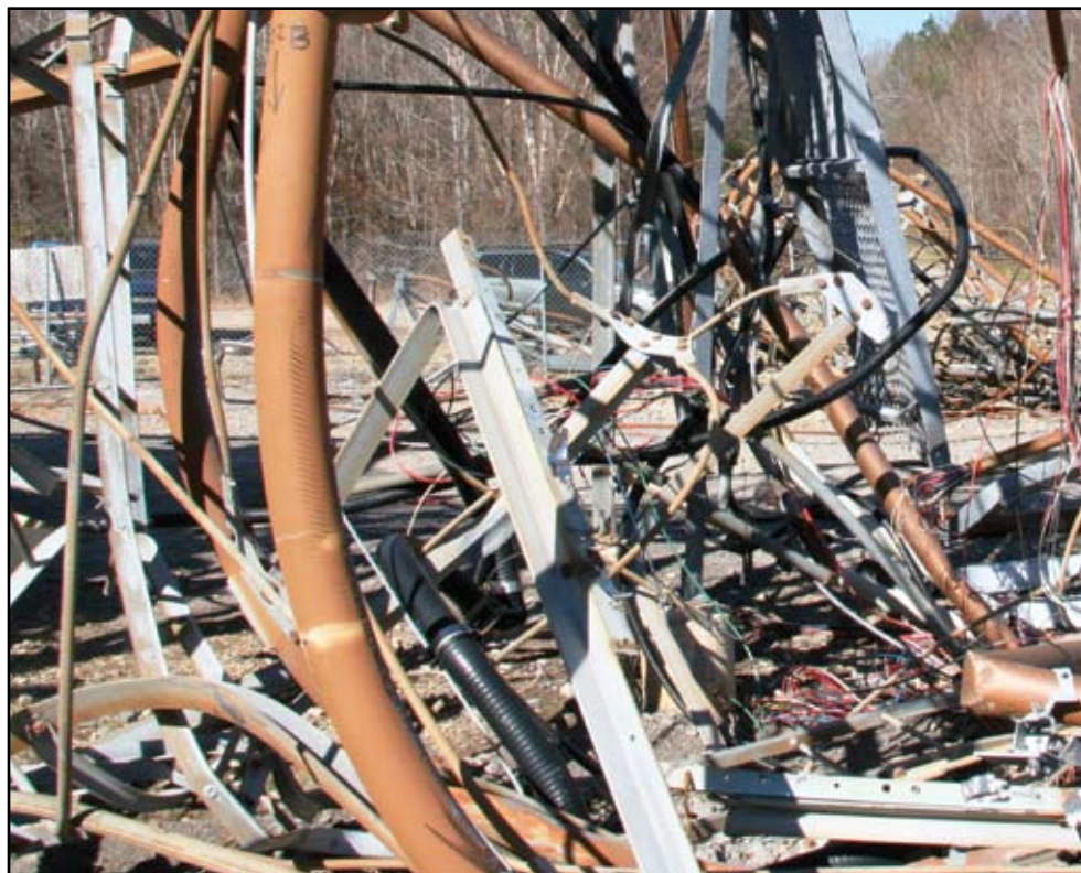
Tower Debris After Failure of a 1000 foot Guyed Tower
