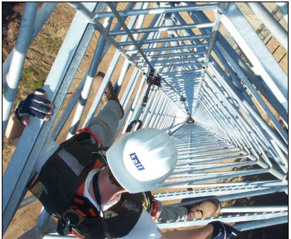
Tower Engineer Inspecting 500 foot Guyed Tower
