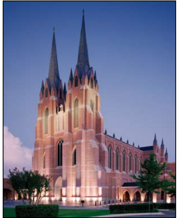
The intricacy of the building's shape, with buttresses, spires, and piers, is true to Gothic precedents. Photo by Mark Scheyer, Inc.
