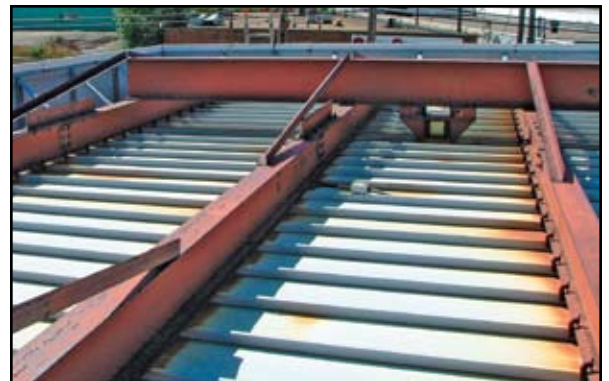
Typical flat canopy framing, ceiling, and fascia panel construction.
