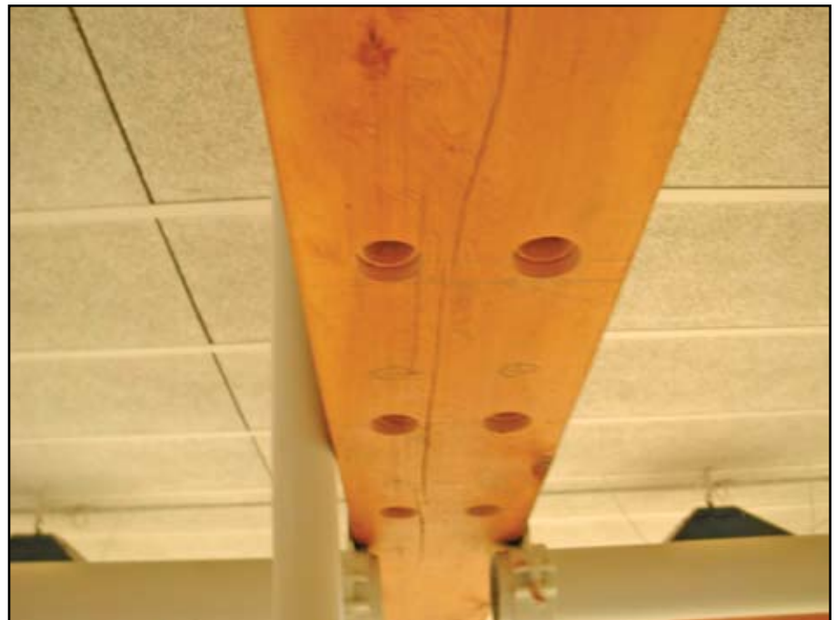
Figure 5: Holes drilled to receive Post-Tensioning Anchor Brackets
