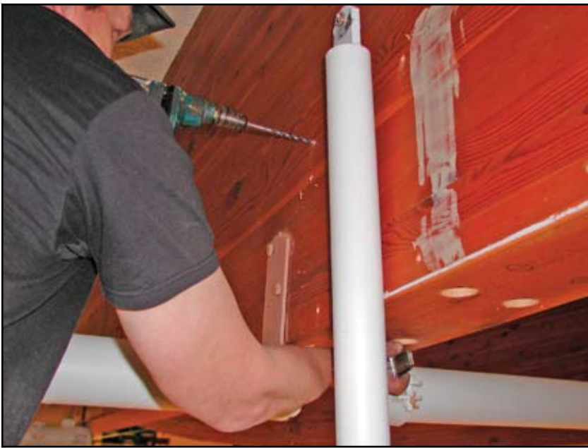
Figure 6: Drilling the injection and exhaust ports
