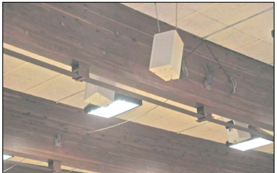
Completed repair/reinforcement of glulam girder beams
