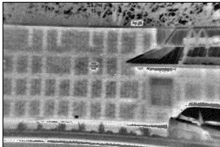
Figure 2: Exterior View of a CMU Wall Taken with an Infrared Camera
