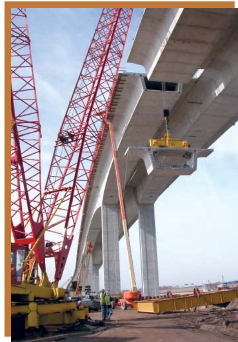
Figure 6: Victory Bridge, New Jersey. Photo courtesy of Figg Engineering Group.
