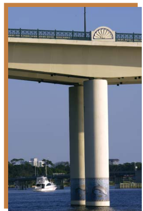
Figure 12: Broadway Bridge in Daytona Beach, Florida. Photo courtesy of Figg Engineering Group.
