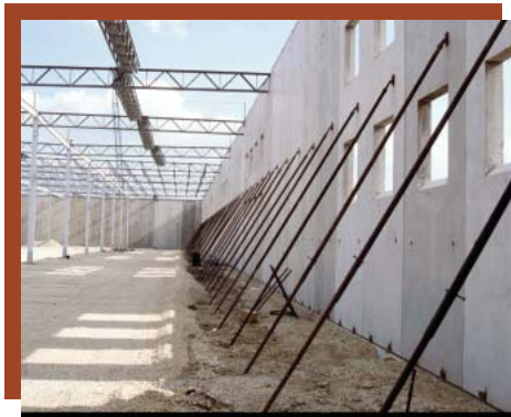
Figure 15: Temporary pipe braces anchored to "Deadmen"
