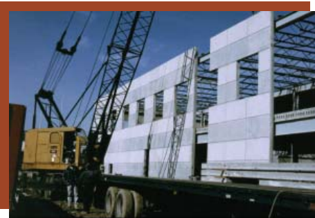
Figure 4b: Non-bearing panels erected at the job site
