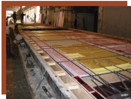
Figure 2: Panels are cast in a long-line form
