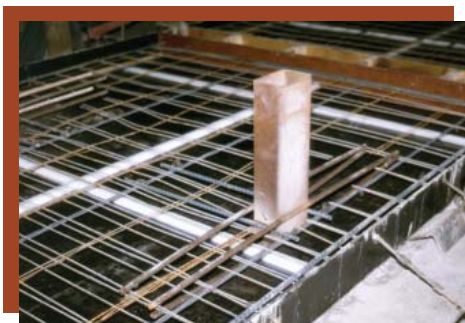
Figure 18: Bearing tube cast into a panel
