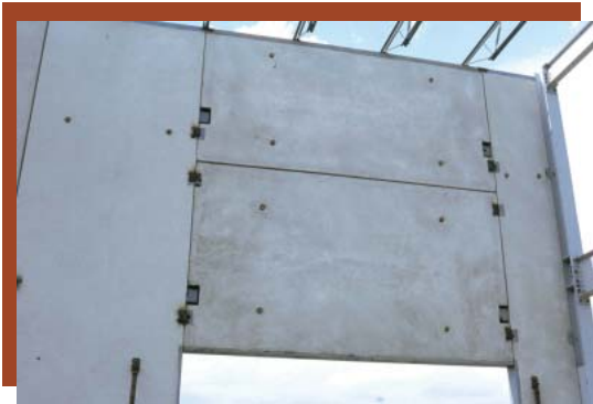
Figure 17: Hung panels supported by bearing tubes & welded plates
