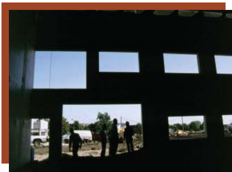
Figure 14: What were they thinking? How not to locate openings
