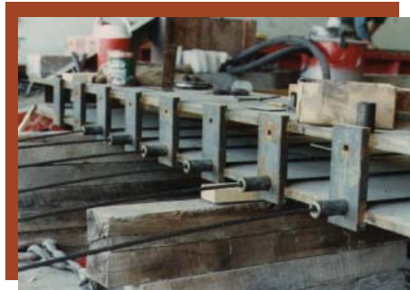
Figure 3: Panels are prestressed
