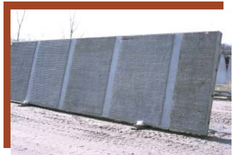
Figure 9: Formliner and reveals used together
