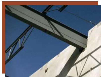
Figure 21: Beam pockets replace exterior columns
