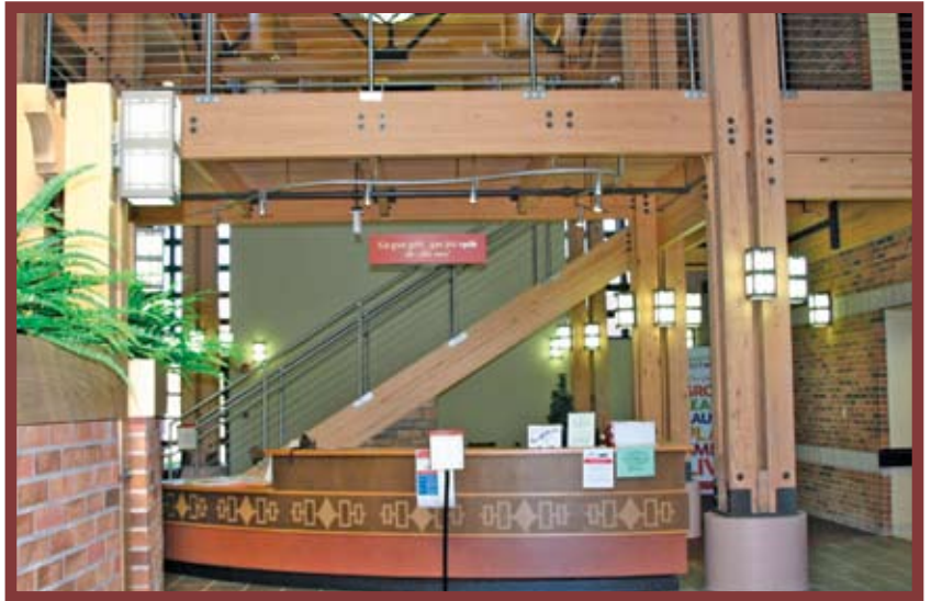
Figure 1: The Seneca Nation Community Health and Wellness Center has an atrium space and multi-purpose room framed with rustic glulam timber.
