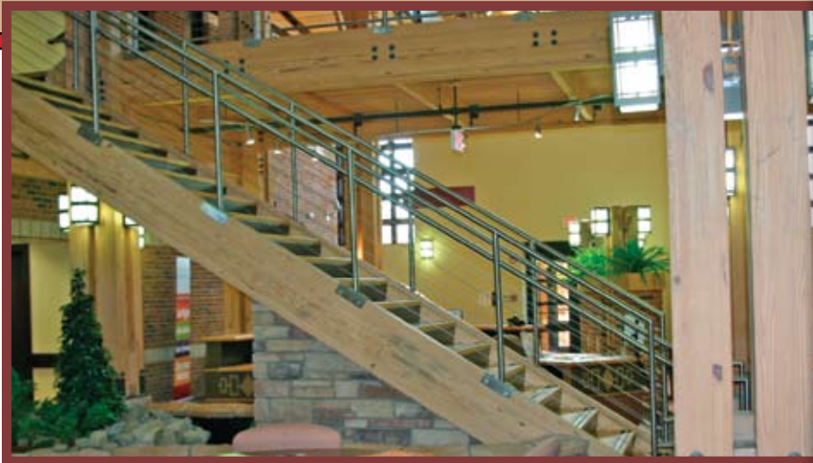
Figure 3: Glulam was also used to construct the stair stringers and "bridge" which spans the atrium, connecting the two office blocks.
