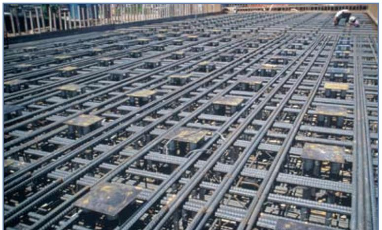
Strong-floor reinforcement layout with anchor point cover plates visible.
