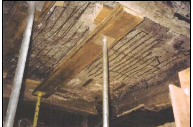
Temporary shoring of the near collapsing cinder concrete slab.
