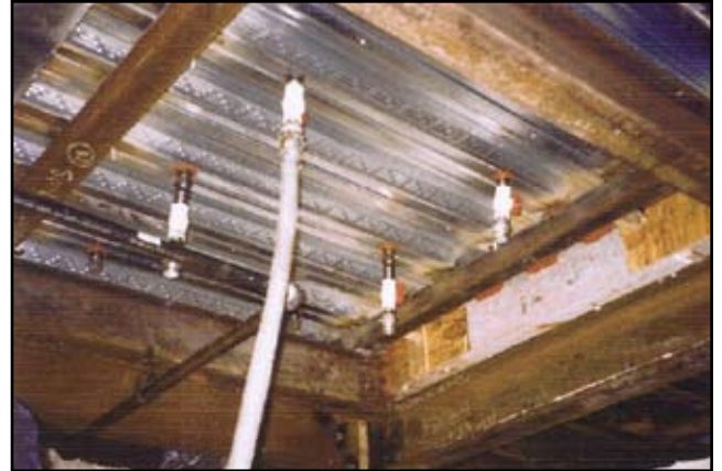
The space between the existing cinder concrete slab and a new metal deck is being grouted. The new deck with injection ports was installed on new sister beams, custom fitted and sealed.
