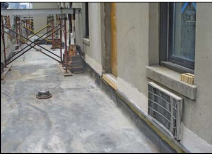
Temporary loose rubber roofing & flashing were installed & new drains added.
