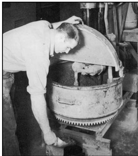
Concrete mixing in the laboratory (from 1951 brochure).
