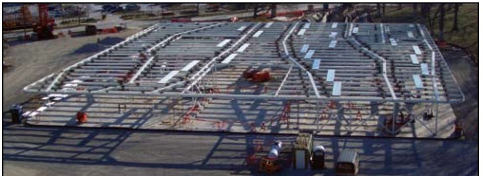
Construction photograph of full steel frame.
