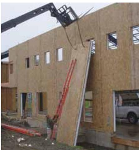
For walls, SIPs provide exceptional strength in racking capacities.
