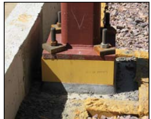
Figure 3: Insulated Column Base to reduce thermal bridging. Courtesy of Russ Miller-Johnson.
