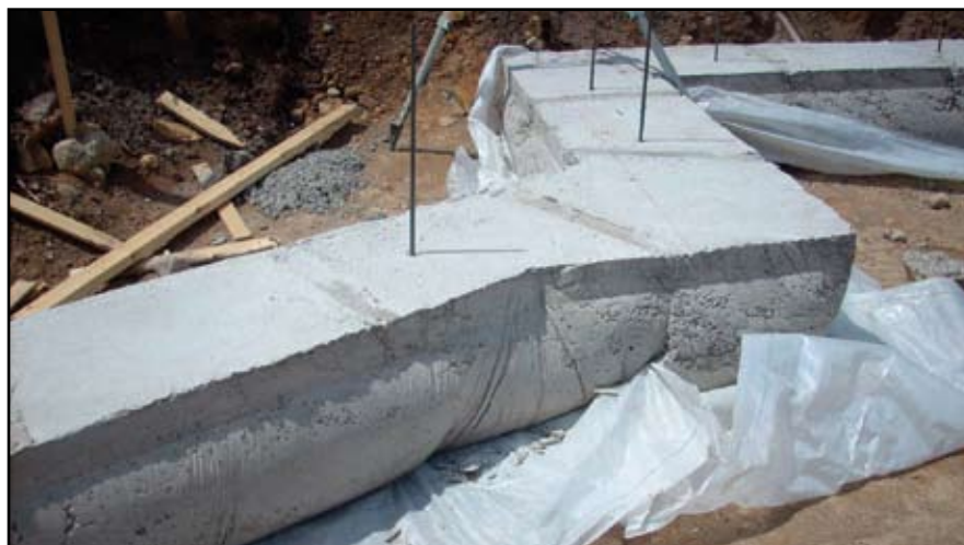
Figure 1: Fabric Formed concrete wall footing. Courtesy of Fab-Form Industries, Ltd ( www.fab-form.com ).
