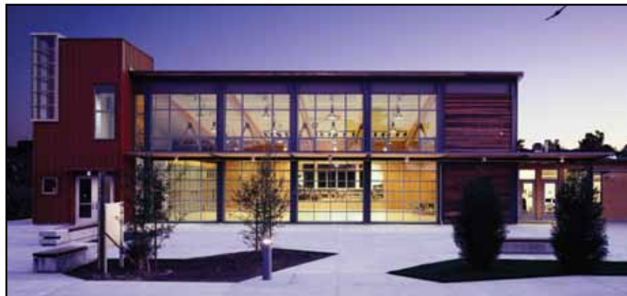
Figure 1: The Chartwell School, Seaside, CA, designed by EHDD Architecture with Tipping + Mar Associates as structural engineer. Courtesy of Michael David Rose / MDRP.NET.
