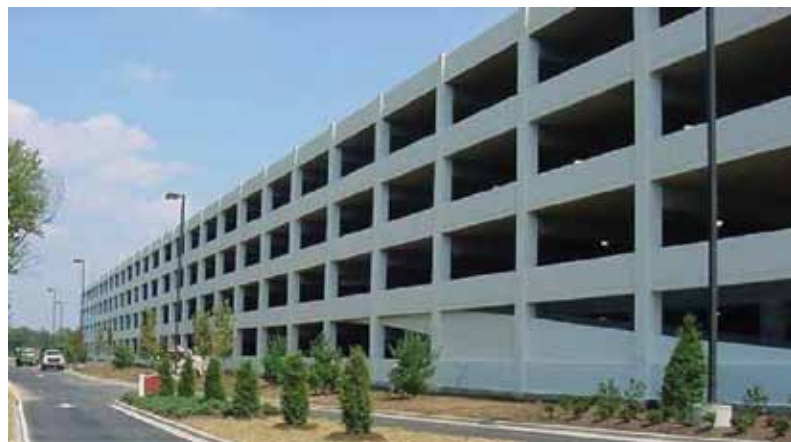
Figure 5: A post-tensioned parking structure in Elizabeth, Indiana with expansion joint spaced at 334 feet (104 meters) apart. (Engineer: Walker Parking Consultants)
