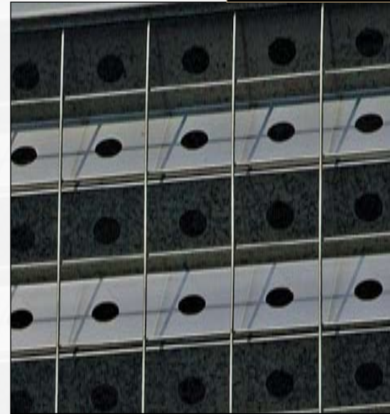
Folded stainless steel guardrail panels with laser cut holes to mitigate headlight glare.
