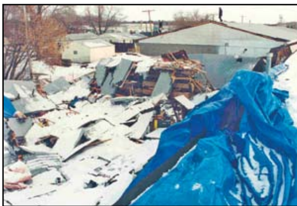
Figure 1: This building roof collapse resulted from a procedural failure in the construction and inspection of permanent bracing, despite the presence of manufacturer-installed red tags shown in the photograph on the right.
