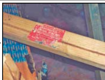
Figure 1: This building roof collapse resulted from a procedural failure in the construction and inspection of permanent bracing, despite the presence of manufacturer-installed red tags shown in the photograph on the right.
