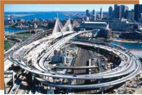
Figure 4: Boston Central Artery/Tunnel, I-93 Viaducts and Ramps. Photo courtesy of Figg Engineering Group.
