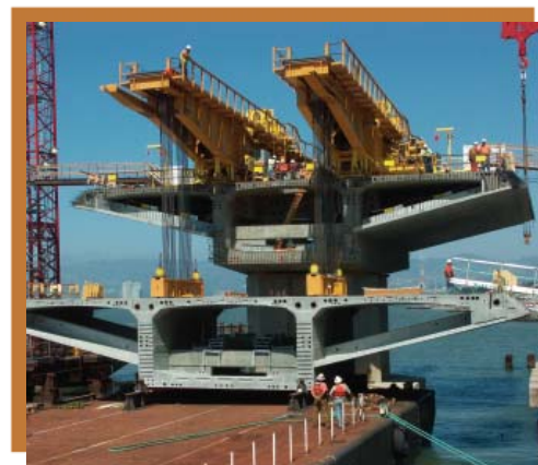
Figure 10: San Francisco-Oakland East Bay Skyway Bridge Segment Erection Device. Photo courtesy of Kiewit/Flatiron/Manson, A Joint Venture.
