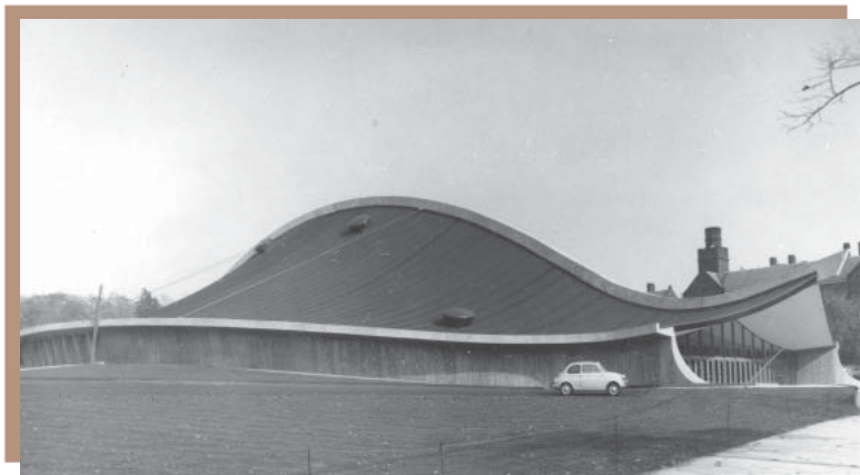
David S. Ingalls Hockey Rink, Yale University, New Haven, Connecticut (1959-61). Its roof structure, 76 feet at its zenith, features two saddle surfaces spanning between three arches. The roof's cable nets are covered with wood decking. Photo courtesy of Fred Severud, Jr.
