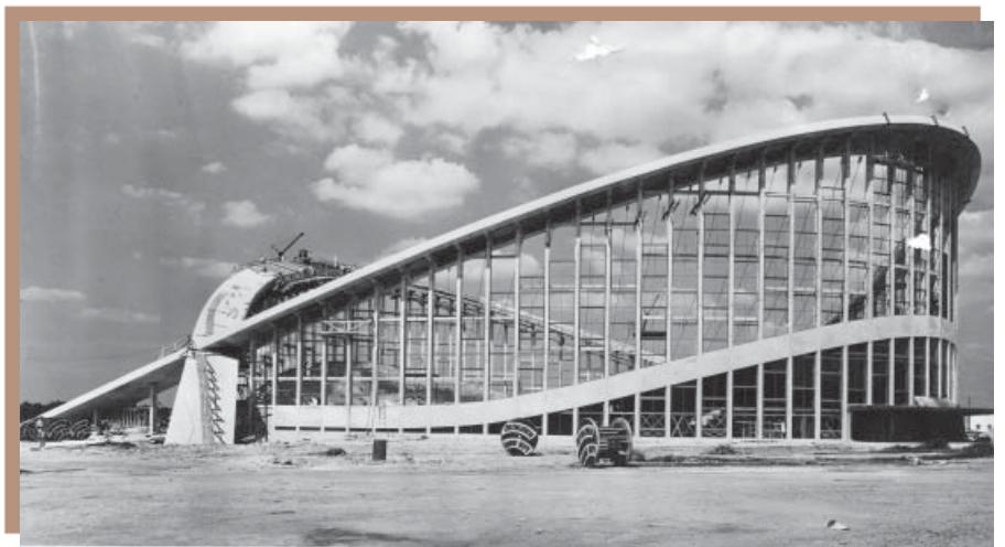
Dorton Arena, the focal point of the North Carolina State Fairgrounds in Raleigh since 1952. Its saddle-shaped, cable-supported roof is supported by wires connected to a pair of intersecting parabolic arches, which are supported on slender columns around the structure's perimeter. Photo courtesy of Fred Severud, Jr.
