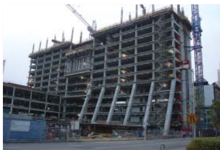
Figure 4: Construction of the San Francisco Federal Building, California (© Arup)
