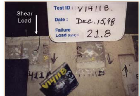
Figure 9: Steel stud failure at a back edge distance of 2½ in. (63.5 mm) or 4d
