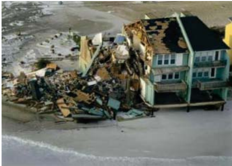
Severe damage to a building is shown in Pensacola Beach, Florida
