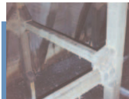
Stacy Park Reservoir Seismic Retrofit 2003 Buildings Under $5 Million Winner
