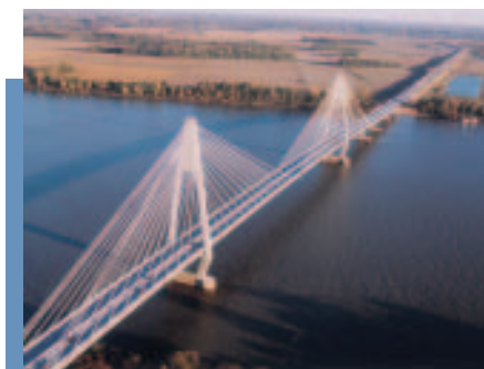
William H. Natcher Bridge 2003 Large Bridge Winner
