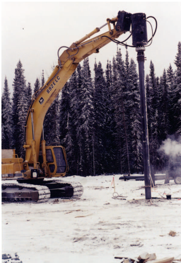
Figure 2: Pile Installation
