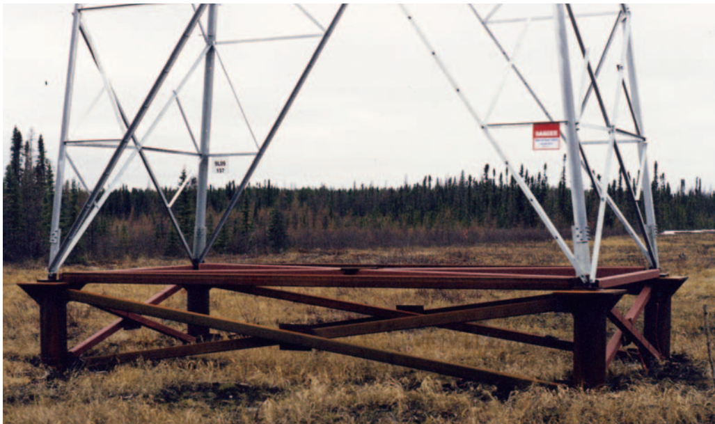
Figure 1: M. Tower Single Pile per leg
