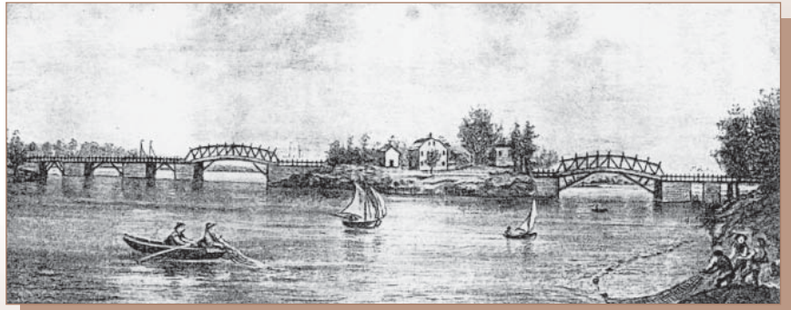
Essex Merrimack Bridge 1792 Looking East
