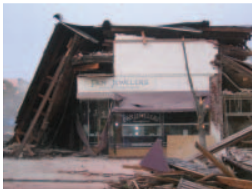
Figure 4 Collapse of the Acorn Building in Paso Robles
