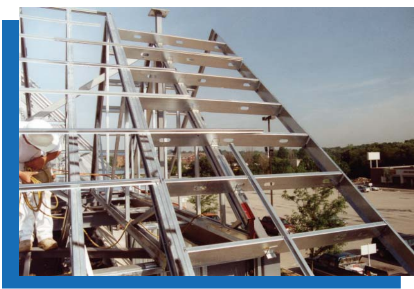
Top Chord Lateral Braces at Gable End
