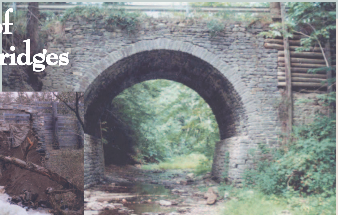
Malta stone arch bridge before collapse
