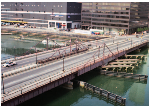
Summer Street slider system bridge
