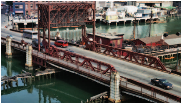
Congress Street bascule system bridge
