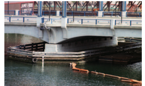
New Northern Avenue Bridge
