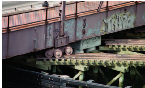
Summer Street Bridge slider system detail
