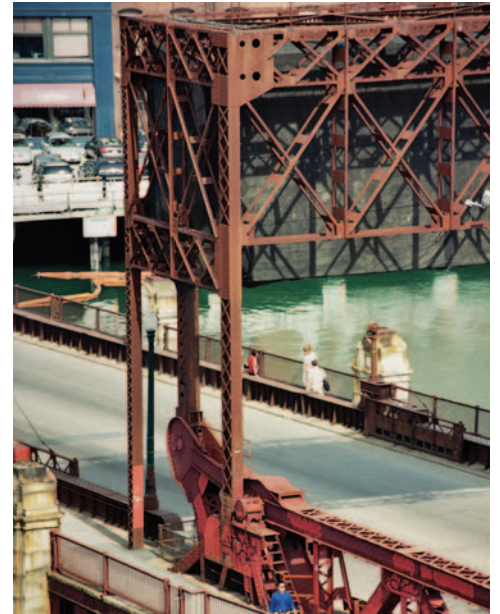
Congress Street Bridge detail of bascule system
