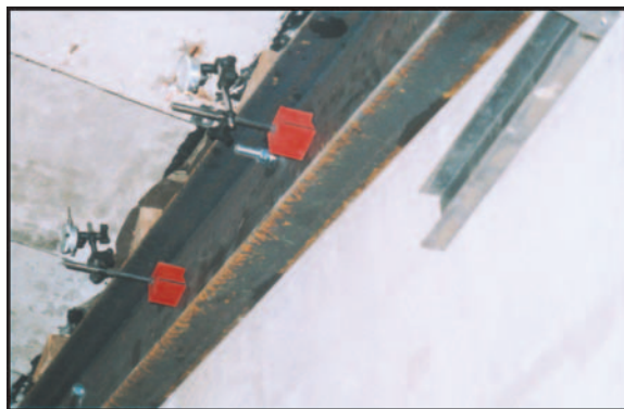
Deflection Measurement During Load Test
