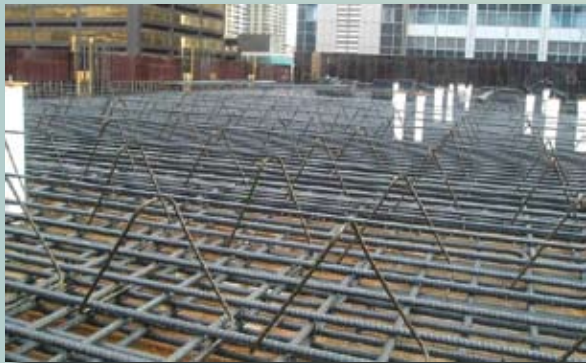
Placement of reinforcement for second lift of transfer mat.
