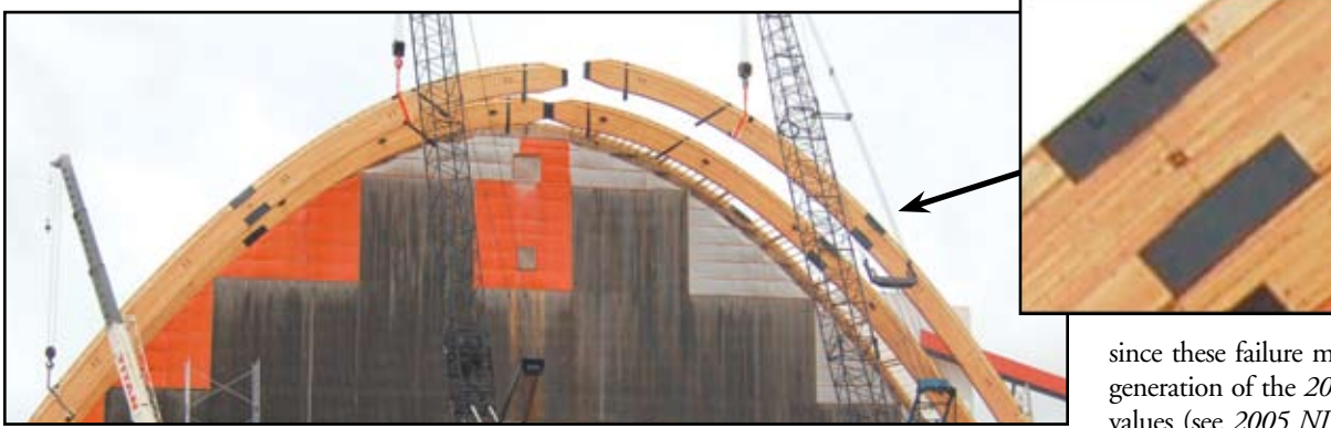
Figure 3: A timber rivet moment splice is part of a three-pinned 12.25-inch x 70-inch 24F-V8 Douglas-fir glulam arch spanning 300 feet.
