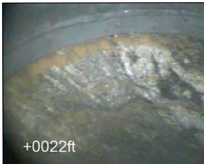
Figure 6: Casing on bedrock.
